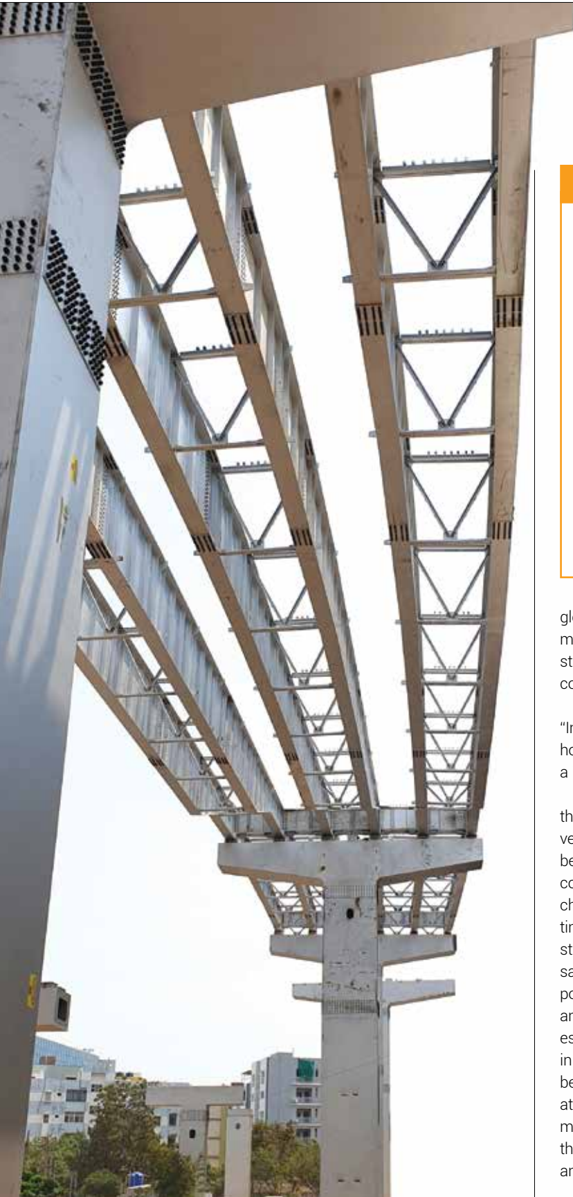
▲ A section of the steel composite bridge under construction.
